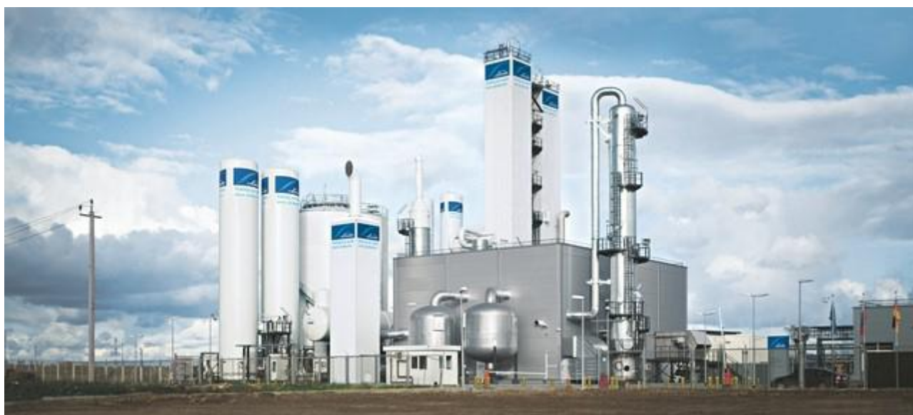
Figure:1 Cryogenic distillation of Air
